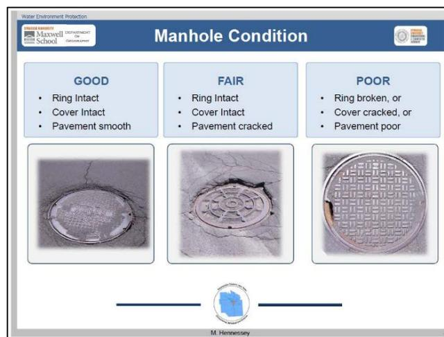
Fig. 4. Manhole Condition Assessment Guide.
