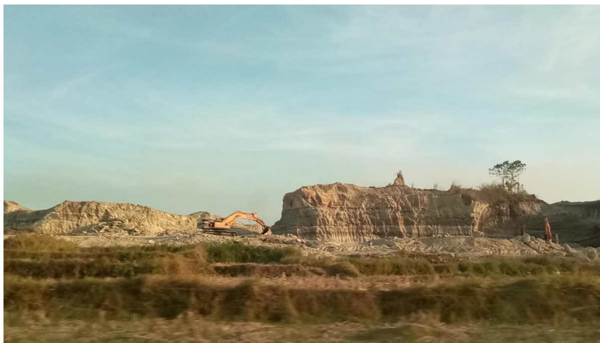
Figure 31. A mountain was excavated to make way for the development of infrastructure in the proposed NCC. This part of a mountain would serve as fillers that would cover what would once be rice fields. Image source: Countermapping Network PH – NCC Research Team
